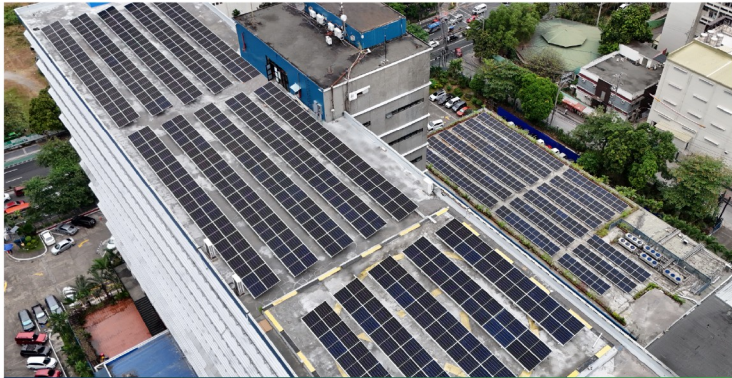
SSS MAIN BUILDING QUEZON CITY
